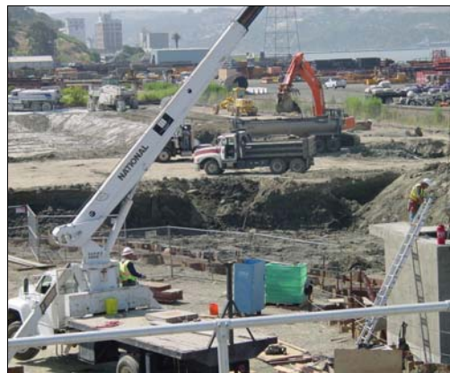
Construction of new 9 million gallon overflow tank.
